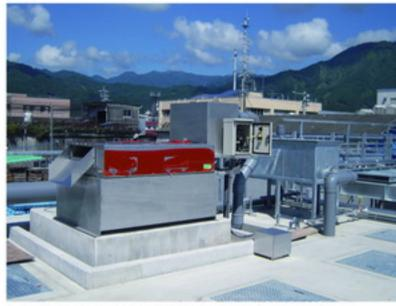
Small-scale demonstration plant for treatment dredged sediments SS-511D
